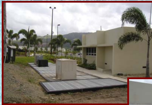
WWTP Project 2003 Industrial
